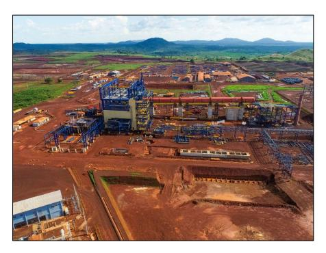
*Figure 3 – A view of the steel erection of the Electrostatic Precipitator, the Rotary Kiln, the Electric Arc Furnace and the Refinery.*
