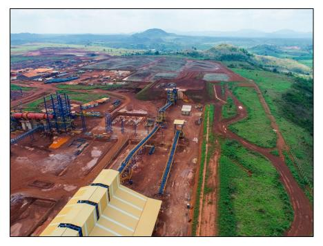
*Figure 2 – A view from above the Homogenisation building looking towards the primary and secondary crushers, the ROM pad and stockpiles.*
