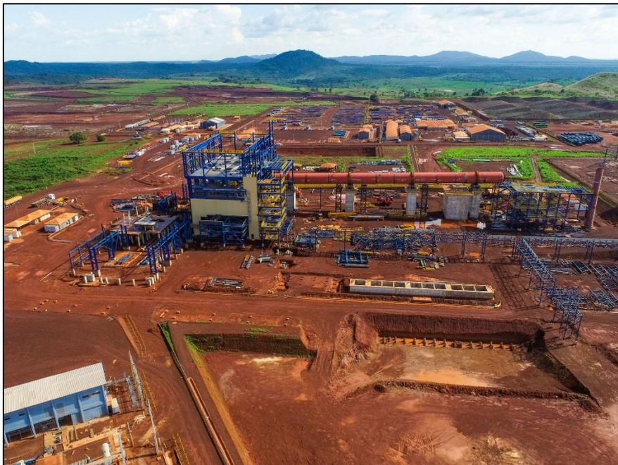
*Figure 3 – A view of the steel erection of the Electrostatic Precipitator, the Rotary Kiln, the Electric Arc Furnace and the Refinery.*
