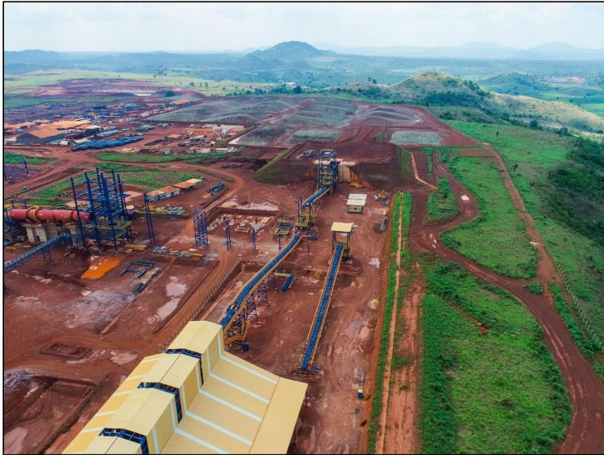
*Figure 2 – A view from above the Homogenisation building looking towards the primary and secondary crushers, the ROM pad and stockpiles.*
