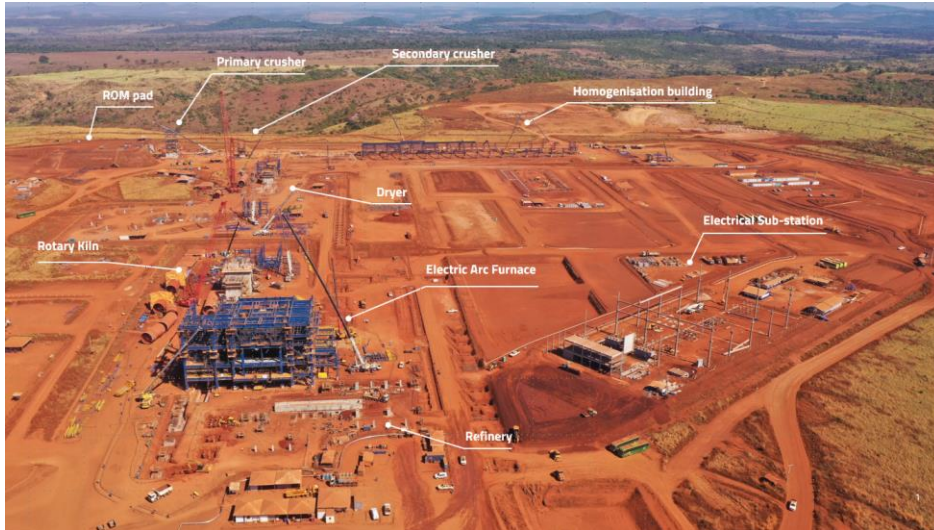
Figure 1 – An overview of the Araguaia processing site
