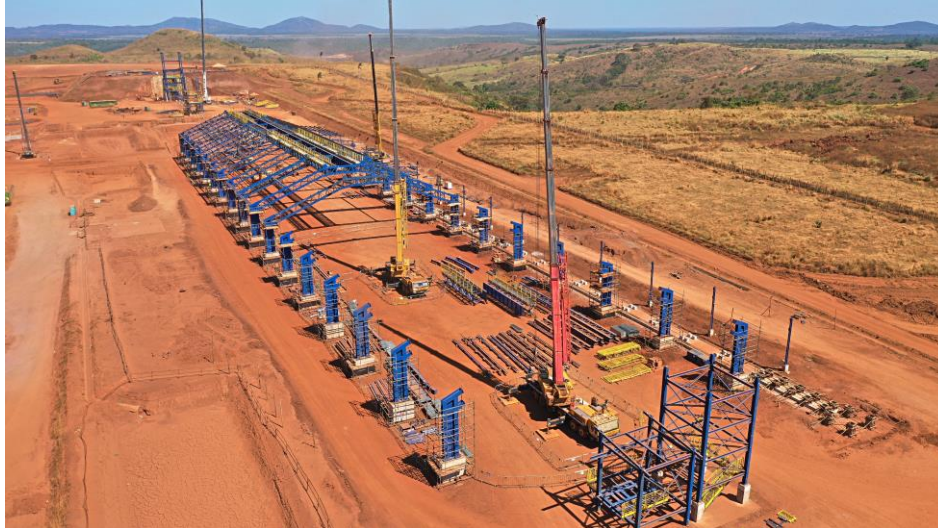
Figure 3 – The Homogenisation shed
