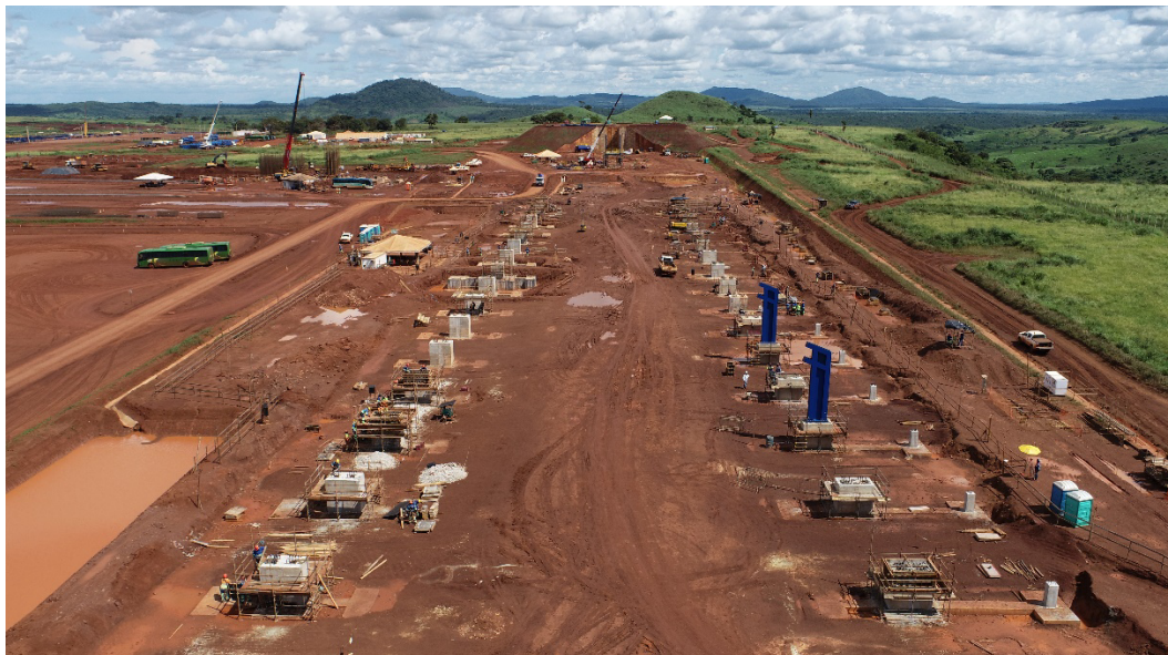
Figure 4: Steel erection works underway on the homogenisation building.
