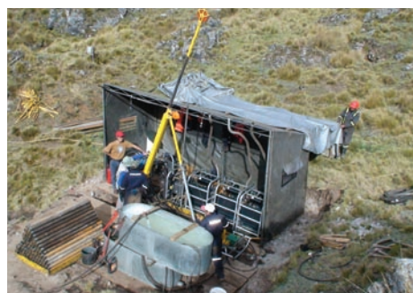
View of drill rig at Zona Sur – El Aguila, Peru
