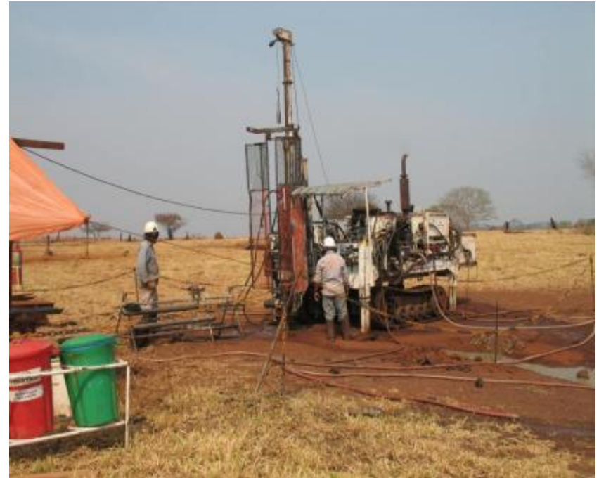
Drilling on the Araguaia project
