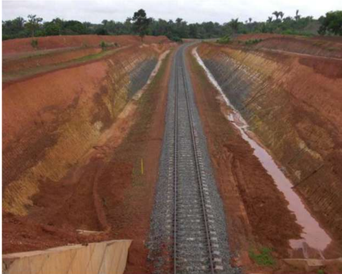
Newly constructed Ferrovia Norte – Sul, west of Palmas, 2011
